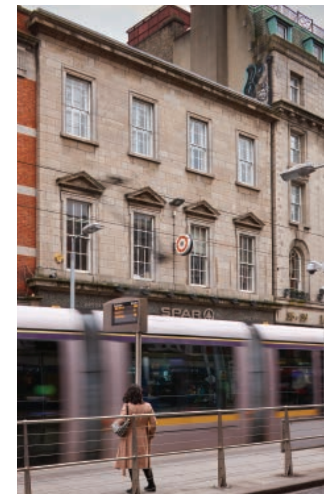
Academy House façade, 2016 IAA survey photograph
