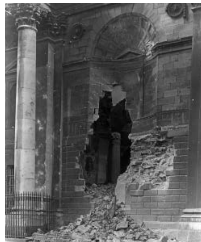
Four Courts, shell damage to front of central block, July 1922 IAA T.J. Byrne Collection, 2012/51.2/350
