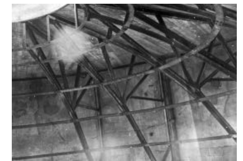
Four Courts, steel support for new concrete dome, 1928 IAA T.J. Byrne Collection, 2012/51.2/53
